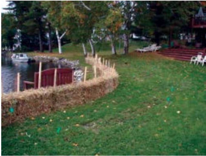
Straw bales protect the water from sediment during a buffer planting.
